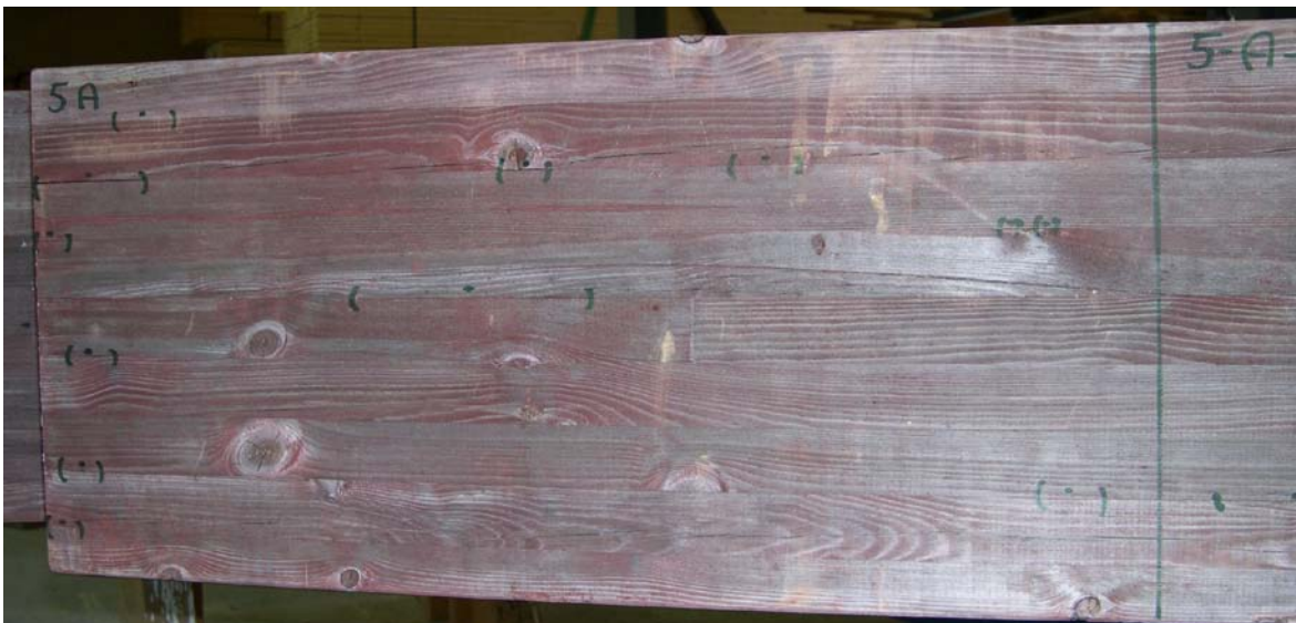
Figure 4.2 Glue line openings – Beam 5A (12,6 %)
