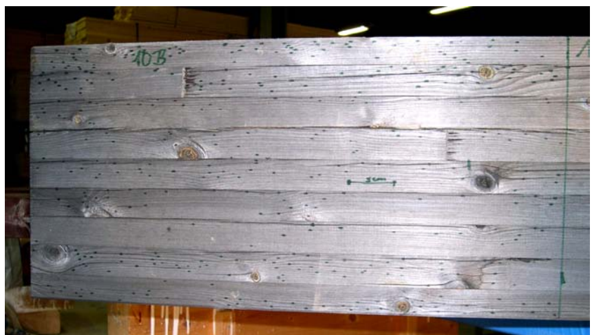
Figure 2.3 Left part of beam 10B with wood cracks
