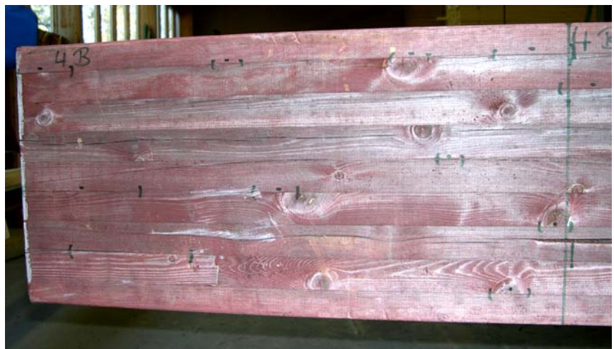
Figure 2.2 Left part of beam 4B with glue line openings
