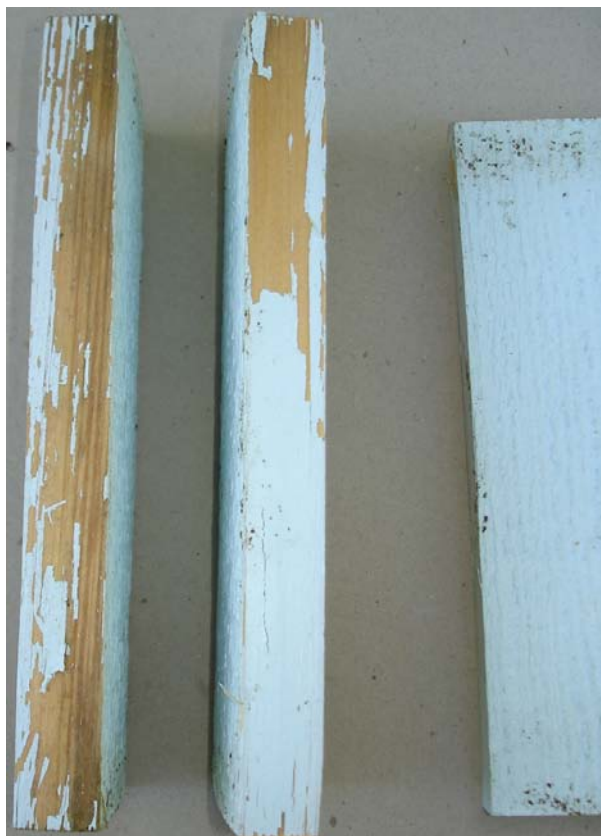
Figure 117. System 9, seen from side.
