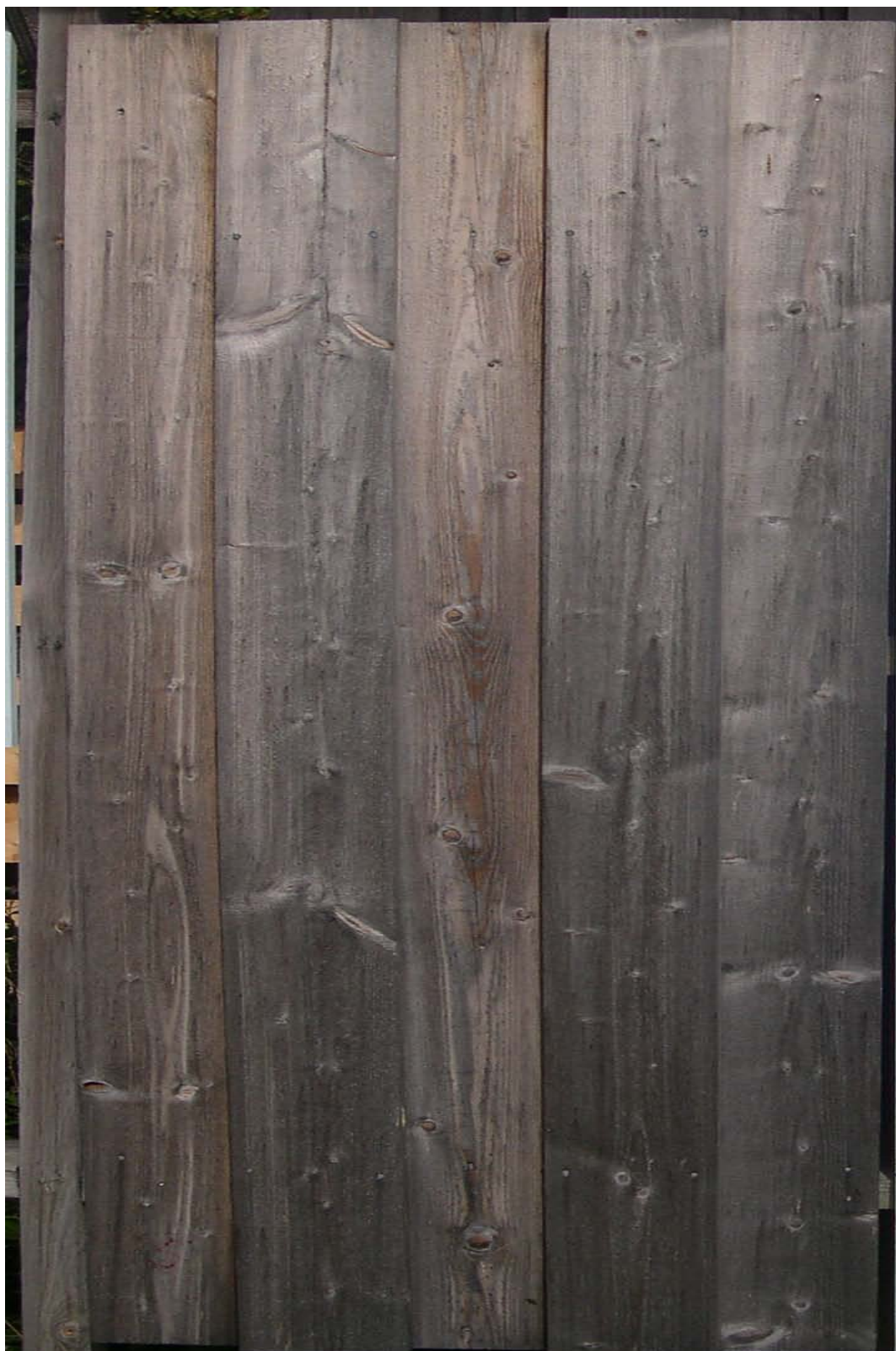
Figur 105. System 15 (ubehandlet gran).
